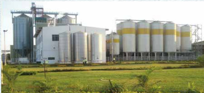
Serengeti Breweries Limited (SBL), has registered tremendous growth in productivity and market value chain, thereby enhancing various stakeholders through direct and in-direct (spin-off effect). Pictured is SBL's Moshi plant, one of the three SBL brewery plants currently undergoing major facelift, including capacity expansion. Other plants are the Dar es Salaam (whose capacity expansion has been completed) and Mwanza plant.
